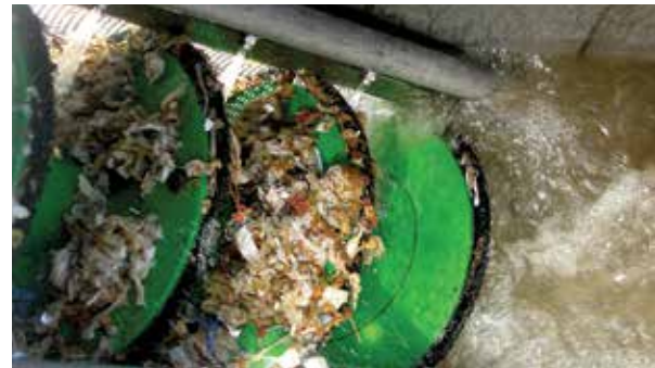
Solids captured and removed by auger
