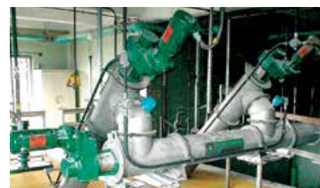
Auger Monsters and cross conveyor
